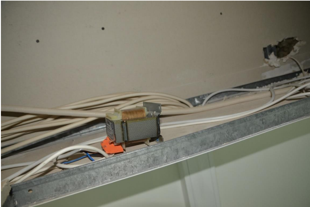
Figure 49: The wiring and transformers' installation
