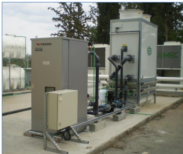
**Figure 32: Absorption chiller and cooling tower**
