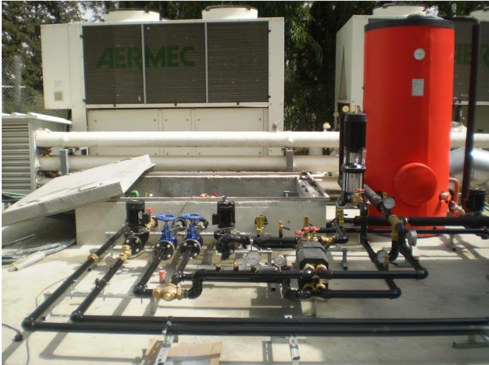
**Figure 30: SHC piping system (integration with HVAC system)**
