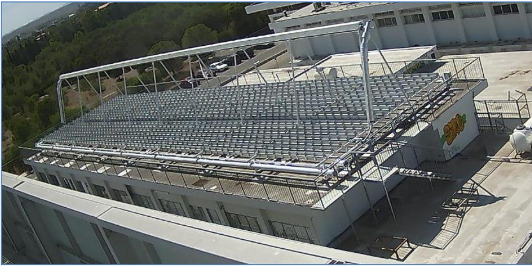
**Figure 26: The Linear Fresnel system installed on the roof of adjacent School**
