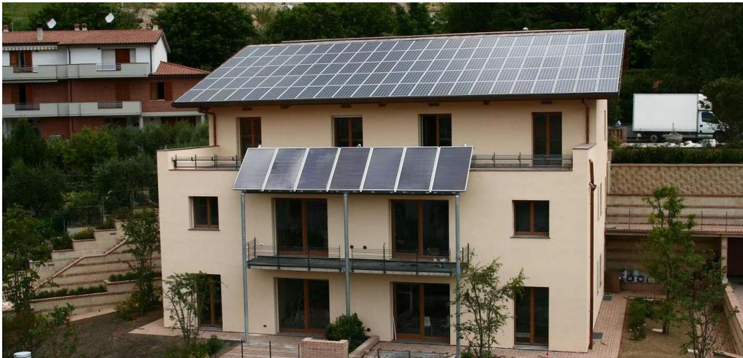
Figure 18: Leaf House building integrated Photovoltaic System (biPV)
